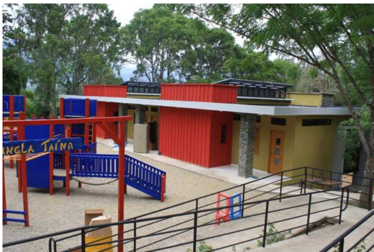
New Elementary classrooms
